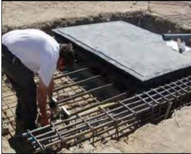
**Picture 6 - Tie down Side Beam Reinforcement**
