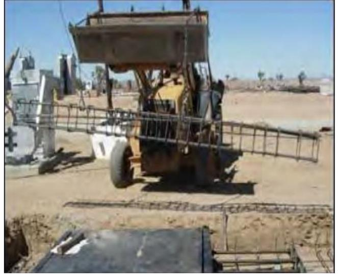
**Picture 5 - Pre-Assembled Side Beam**
