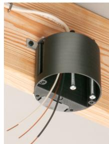
**3** Pull NM cable through installed NM connector.
