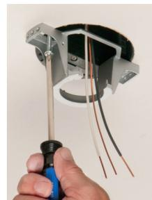
**6** Box flush with ceiling. Remove captive installation screws and install bracket.
