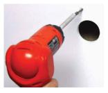
Orill holes into the drywall and insert the drywall mounts into the holes.
