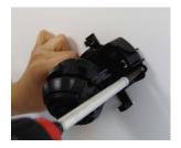
Pull wires through and make connections. Then, mount the camera to the wall using the included machine screws
