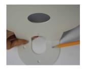
② Use the mount to mark the pilot holes that are required. Drill holes into the drywall and insert the drywall mounts.
