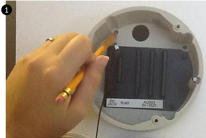
1. Use the camera's mounting template or your camera to mark the holes as required.
