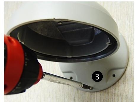
3. Use the mounting template to make pilot holes. Use the dry wall anchors and wood screws to attach the assembly to the wall.
