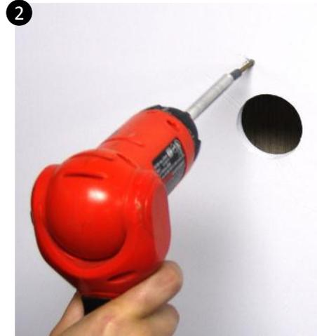
2. Drill holes into the drywall and insert the drywall mounts into the holes.
