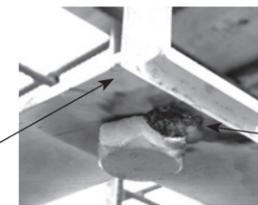
**6** Ensure anchor cage location is maintained while pouring the concrete. **Tip:** Tack weld bolt heads to base of anchor cage (10x). DO NOT weld to the round shank of the bolt.
