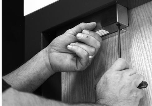
Figure 17. Installing the Magnalock
