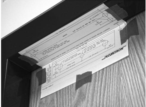
Figure 4. Attaching the Template
