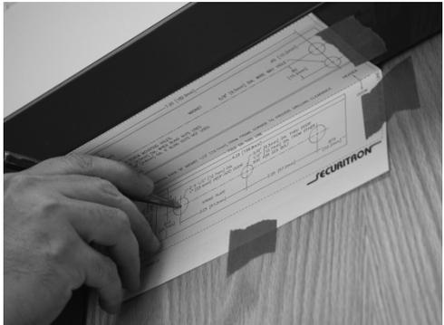
Figure 5. Marking Drill Hole Locations
