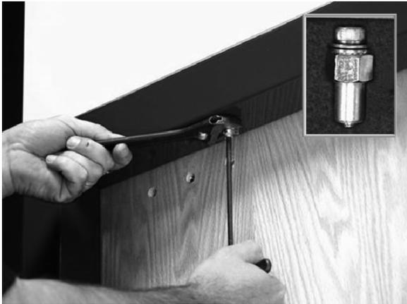
**Figure 9. Installing the Blind Nuts**
