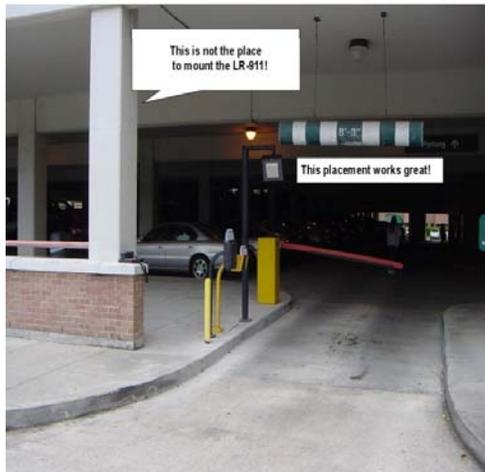
In this instance, the fact that vehicles were turning through the read zone meant poor performance when the reader was mounted on the white post. Once the reader was moved back closer to the operator, it worked much better!
