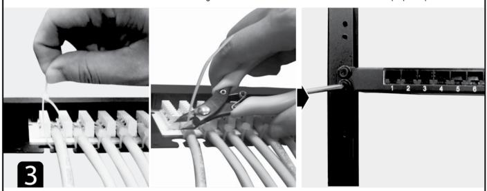
Secure the bulk cables to the cable manager using nylon cable ties. (Note: please do not over-tighten the cables.) And, cut off all the excess straps. Fix the terminated panel on the rack.
